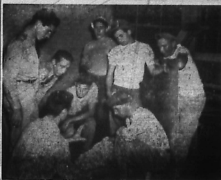
CONSULTING FLOAT BLUEPRINTS just before they begin construction are, left to right, Yalton Holley, Ken Evans, Charles Eastman, Billy McGee, David Phillips, Jerry Shields, Tommy Latimer and Jack Poole.
