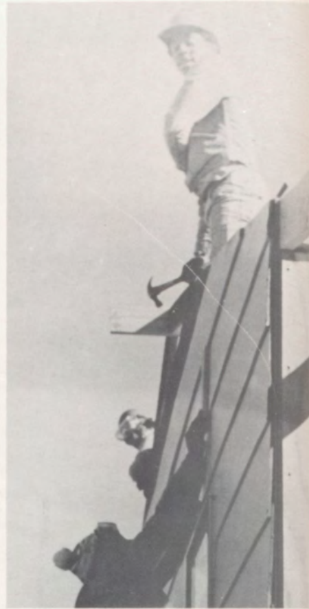
Students work on the house.
