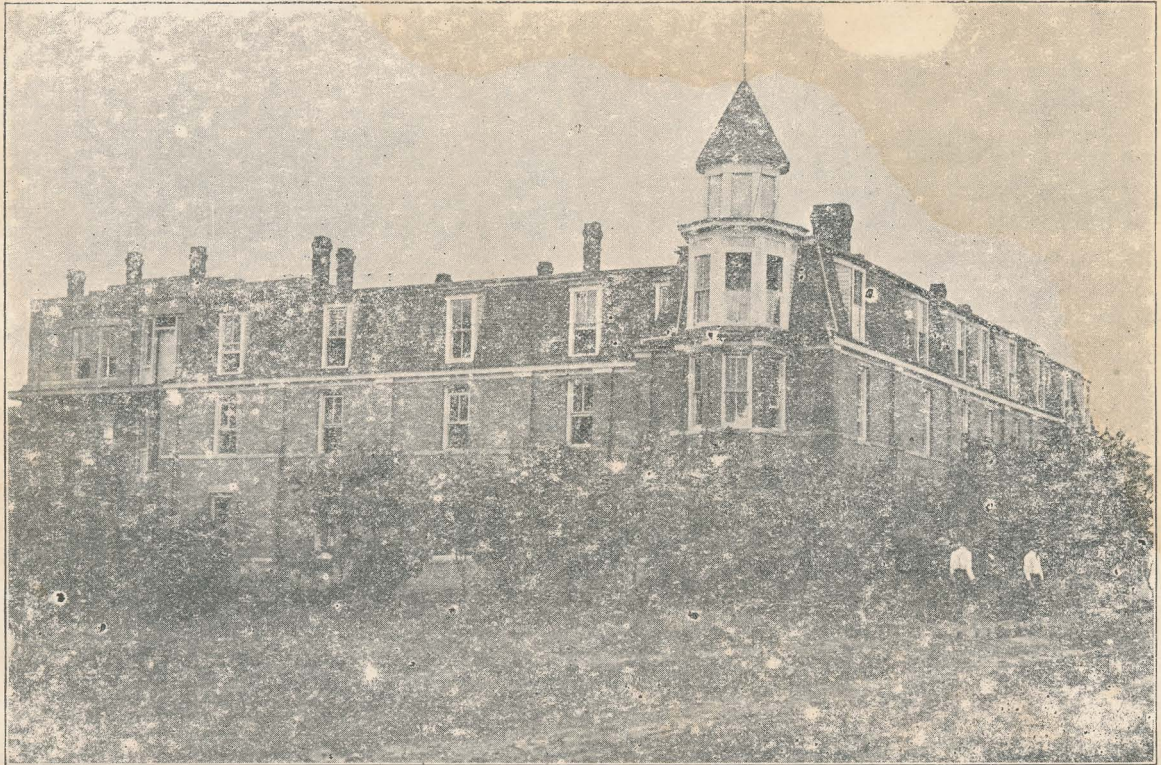
DORMITORY FOR MEN
